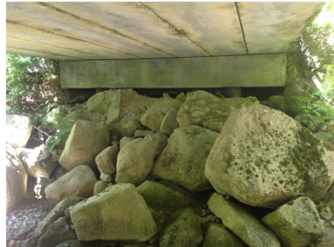
Right Bank Abutment when facing downstream
