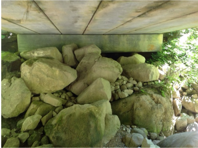
Left Bank Abutment when facing downstream
